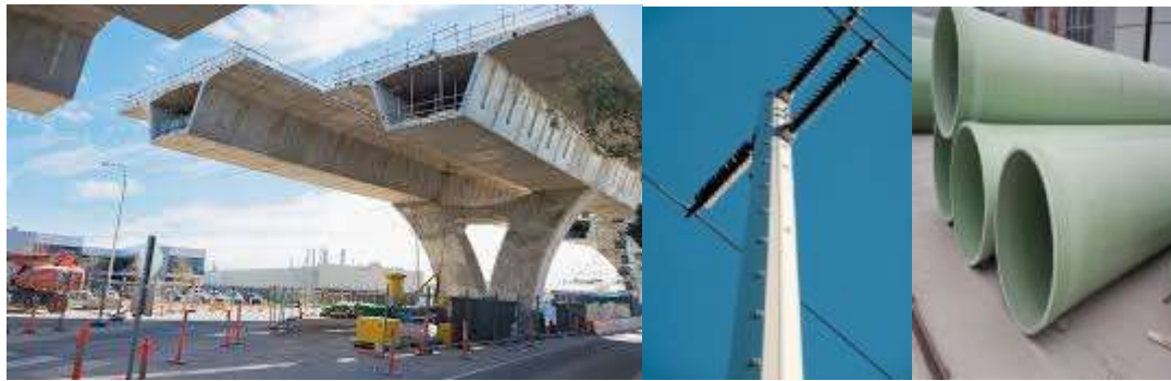
Figure 3: applications of fiber reinforced composites in (a) pedestrian bridge construction (Moore, 2019) (b) Utility pole in-service (GangaRao, 2011). (c) Water and Oil transportation
