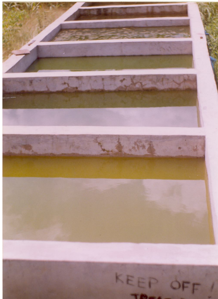
Plate 1b: Photograph showing the flooded and treated ponds
